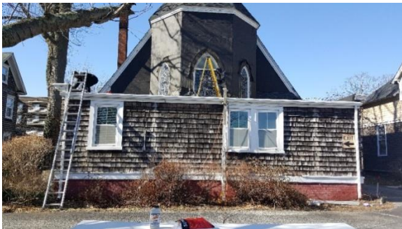
Repairing the leaking roof of long standing!
